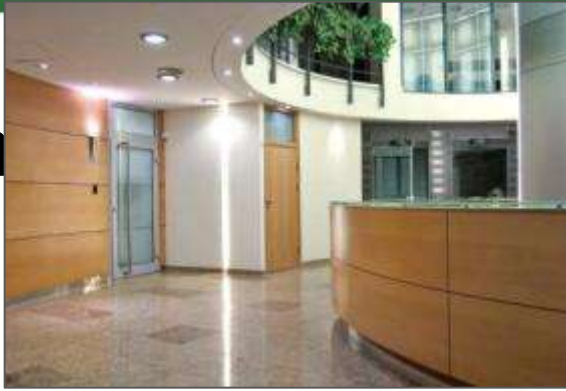
Track & Recessed Lighting
